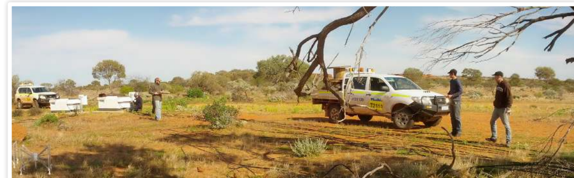
Figure 3: Laying cables in the unusual green desert.
